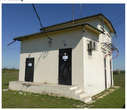
**High voltage laboratory** is in the same area like Varna South substation. This is the only one certified high voltage laboratory for Bulgaria. High voltage generators 2,000 kV and 700 kV are installed. Isolators and other parts for distribution are tested here. Also training classrooms are present here. Administrative building is situated in the same area.
