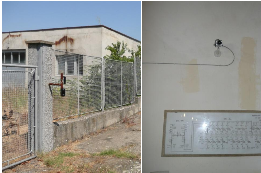
Picture 12: Infrared gates and CCTV
